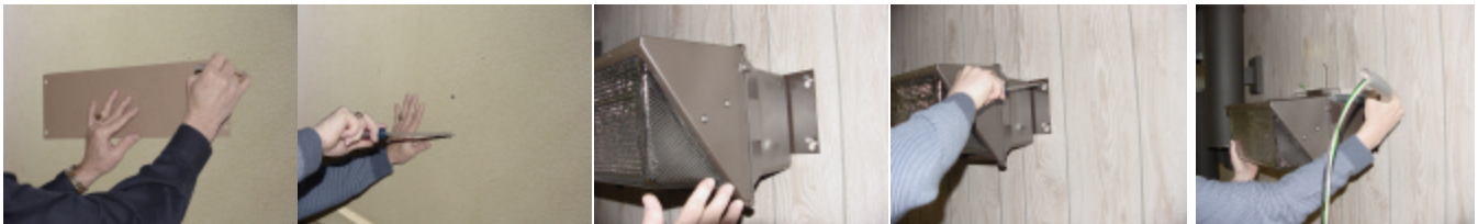
STEP 1. Mark wall with supplied template.
