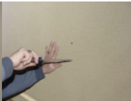
STEP 2. Start fasteners in wall.
