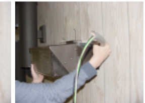
STEP 5. Connect wall pack external j-box.
