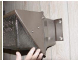
STEP 3. Hang wall pack using keyhole slots.
