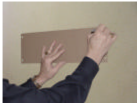
STEP 1. Mark wall with supplied template.
