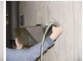
STEP 5. Connect wall pack external j-box.
