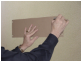
STEP 1. Mark wall with supplied template.
