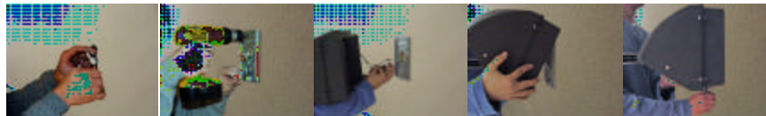
STEP 1. Connect quick connector to power supply. STEP 2. Attach cast aluminum mounting plate on recessed j-box. STEP 3. Connect quick connector from power source to fixture. STEP 4. Hang wall pack on mounting plate. STEP 5. Secure wall pack to mounting plate with locking screw.
