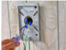
STEP 2. Attach cast aluminum mounting plate on recessed j-box.
