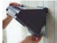
STEP 4. Hang wall pack on mounting plate.
