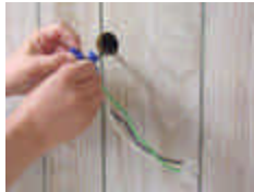
STEP 1. Connect quick connector to power supply.
