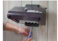
STEP 5. Secure wall pack to mounting plate with locking screw.
