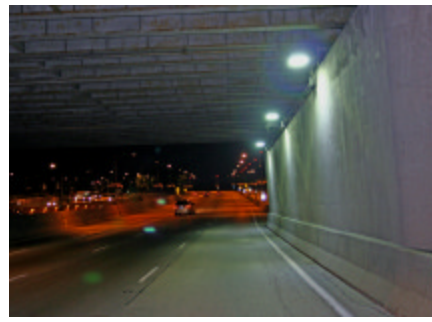
After: Energy efficient 120 watt Esco LED tunnel fixtures. Bright white light LEDs create excellent color rendering (80 CRI).
