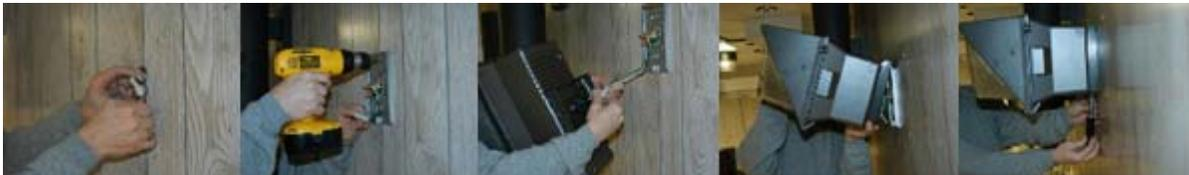
Step 1. Connect quick connector to power supply.
